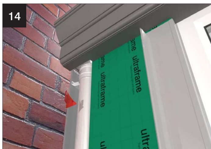
Fit concealed rainwater downpipe (if ordered)
