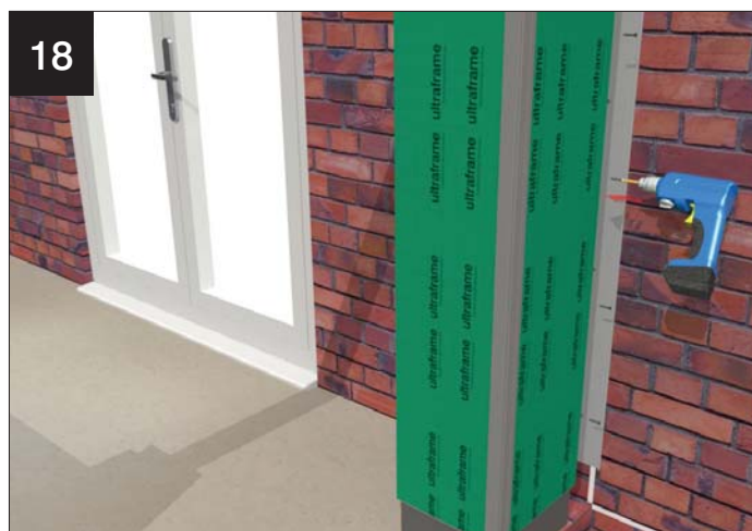
18 If an abutment is specified, permanently fix the column to the wall bracket using the screws supplied as shown (4.8 x 25mm pozi pan head self tap screw).
